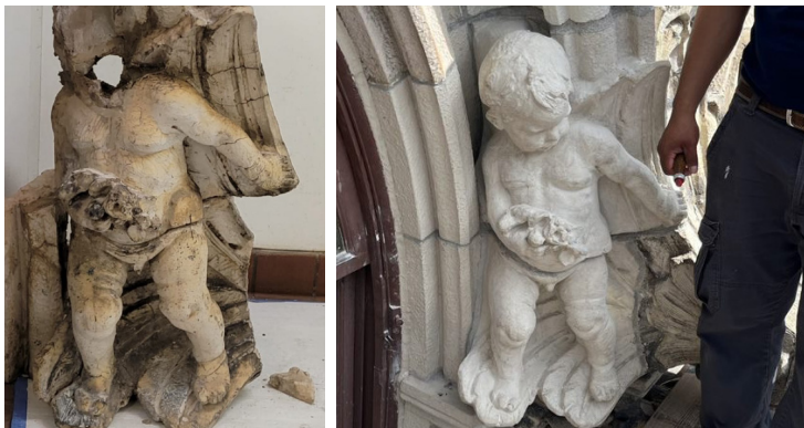
Original sculpture (left) and a Vestacast replica (right) at the Croisic Building. The company also produced the replicas (top) at the Fifth Ave. landmark.
