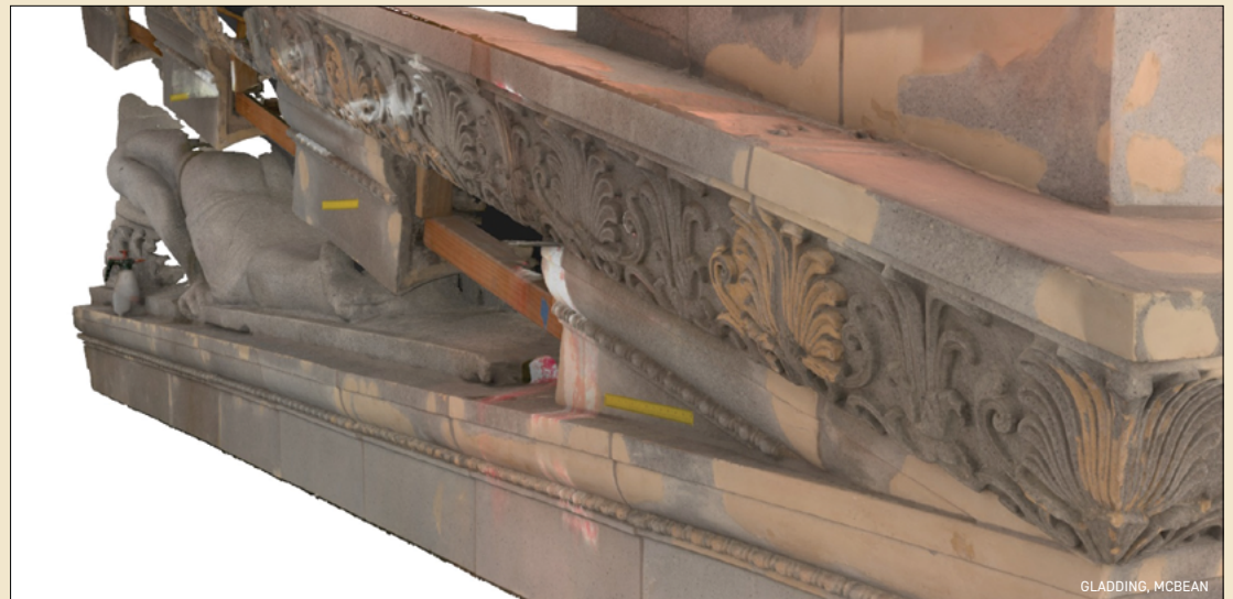
Above: A member of the Gladding, McBean Drafting and Survey Team operating a handheld scanner at a jobsite. Below: The 3D model created directly from the scans gathered in the field.
